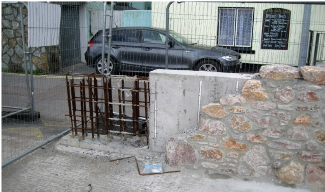
Photo 5.1 - Reinforced concrete flood resistant wall faced with local stone © Robin Stott
